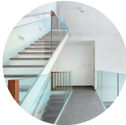
All Winstone Glass balustrades are designed to meet the new safety standards. For balustrades and deck enclosures, toughened or laminated safety glass provides a functional barrier that is also easy on the eye. Panels can be shaped, frosted, coloured or screenprinted to add extra personality to your surroundings. All the exposed edges of the glass are polished for safety to give them a fine quality finish.
